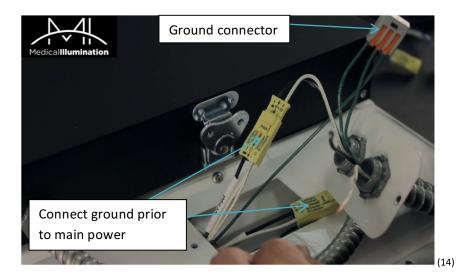
Remove the male portion of the power connectors and connect one to each of the incoming power circuits. (Image 15)
